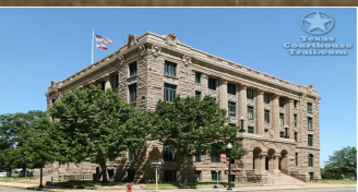
Lamar County Court House
