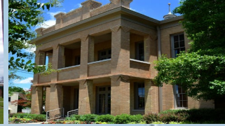
Morris County Court House
