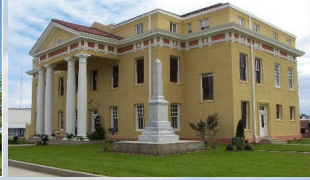
Cass County Court House
